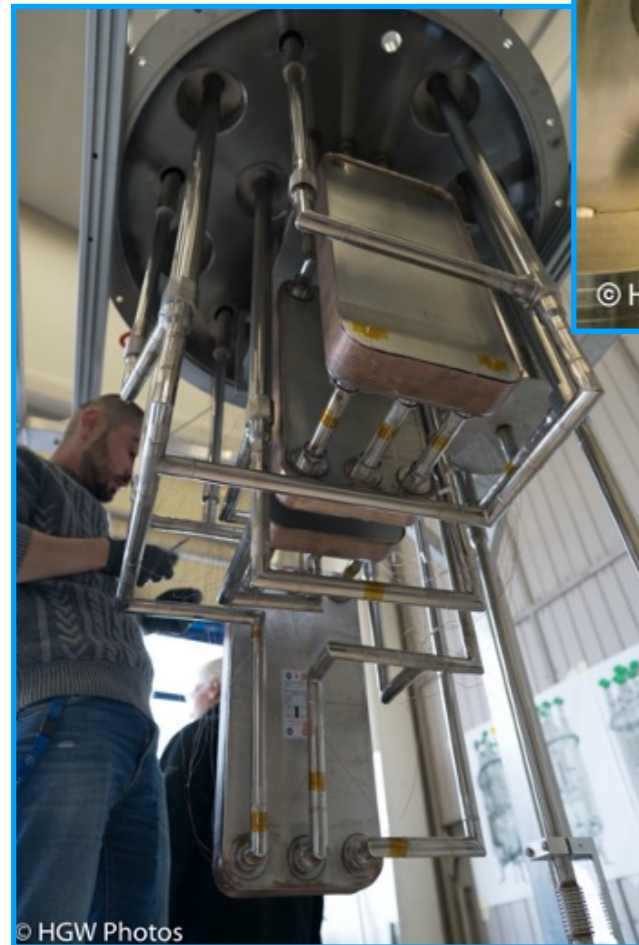
In-house fabrication of the gas handling system
